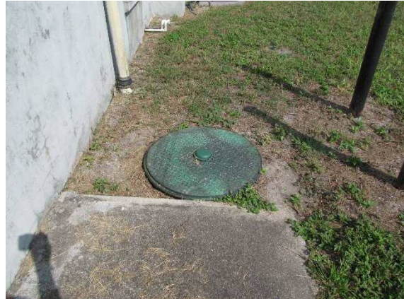
Sewer connection SW corner of building
